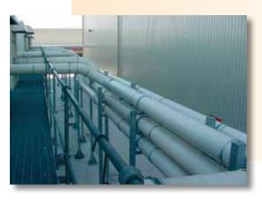
Supplied in flanged or clamp lengths, long radius bends to reduce friction, various materials of construction are available to suit chip type. Surface finish to customer specification.
