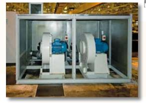
Heavy duty centrifugal type fan units housed in attenuated enclosure and having energy efficient drives and automatic run & standby changeover facilities.
